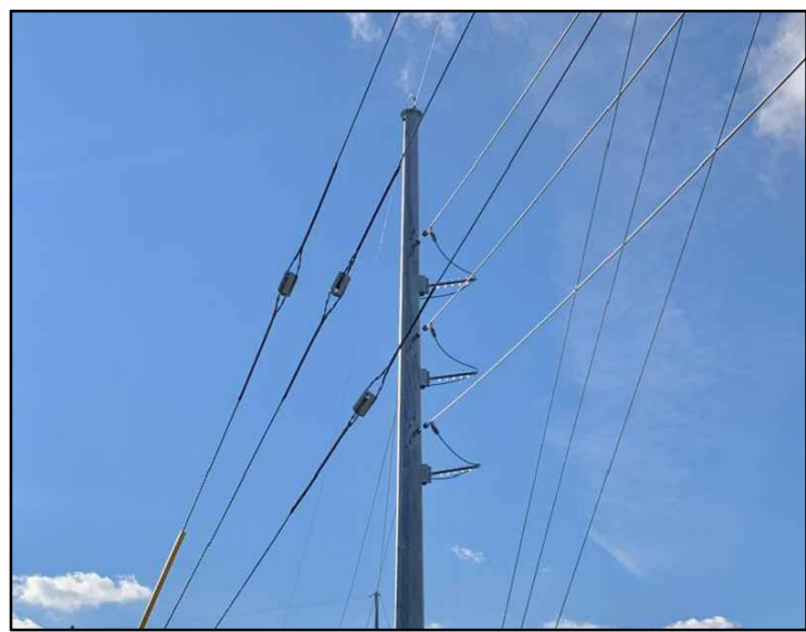
SELF SUPPORTING STEEL MONOPOLE
