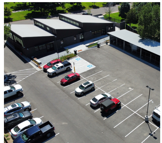
Completed Rosedale Maintenance Facility.
