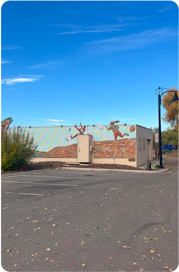
Existing Pump House Area
