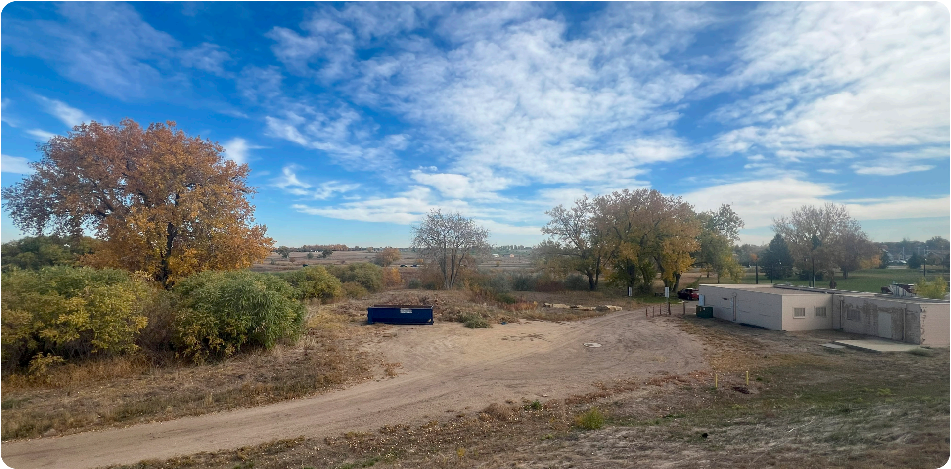
Existing Pump House Area
