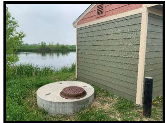
Centennial Park Pump House
