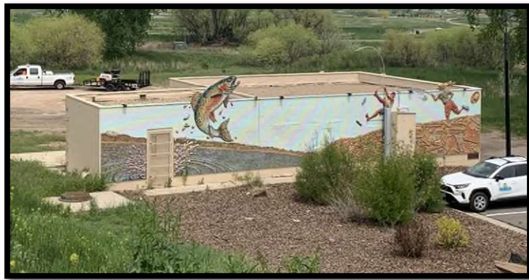
East Milavec Pump Station
