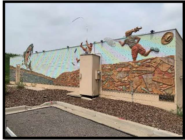
East Milavec Pump Station
