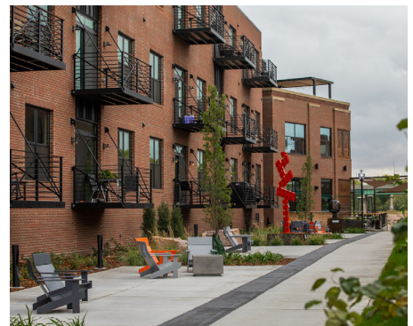
Picture of an urban apartment complex. It has red brick with metal balconies, with room for lawn chairs in the foreground. Credit: Shutterstock
