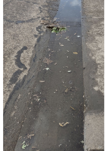
Gutter nuisance flow
