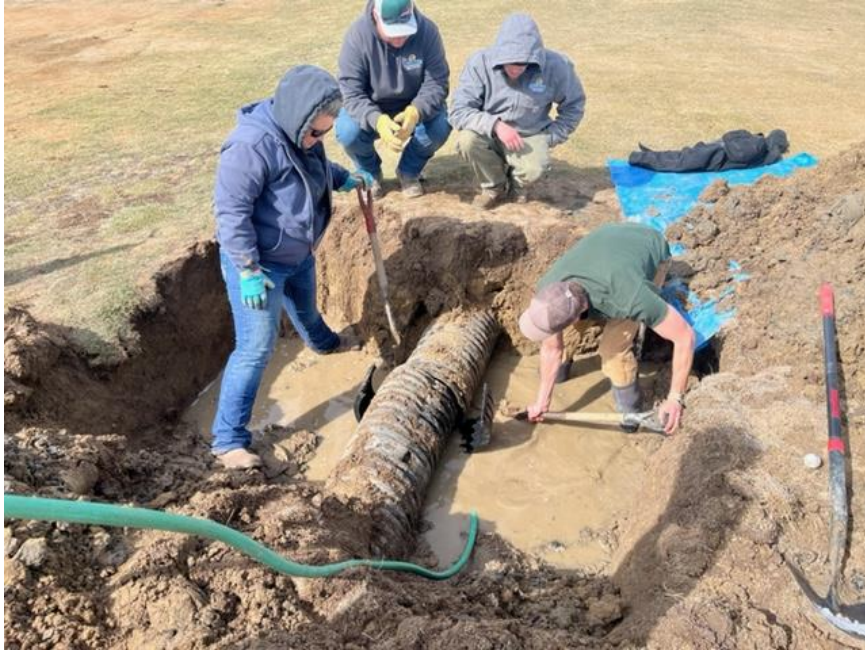
Early season drainage pipe repair project. The Parks staff assisted in digging & repairing a 12 inch drain pipe.
