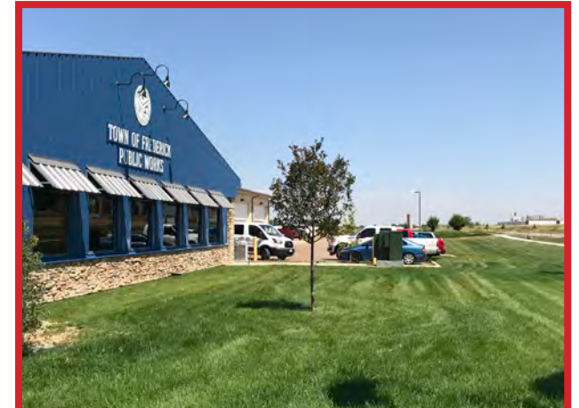
Lack of Shade
