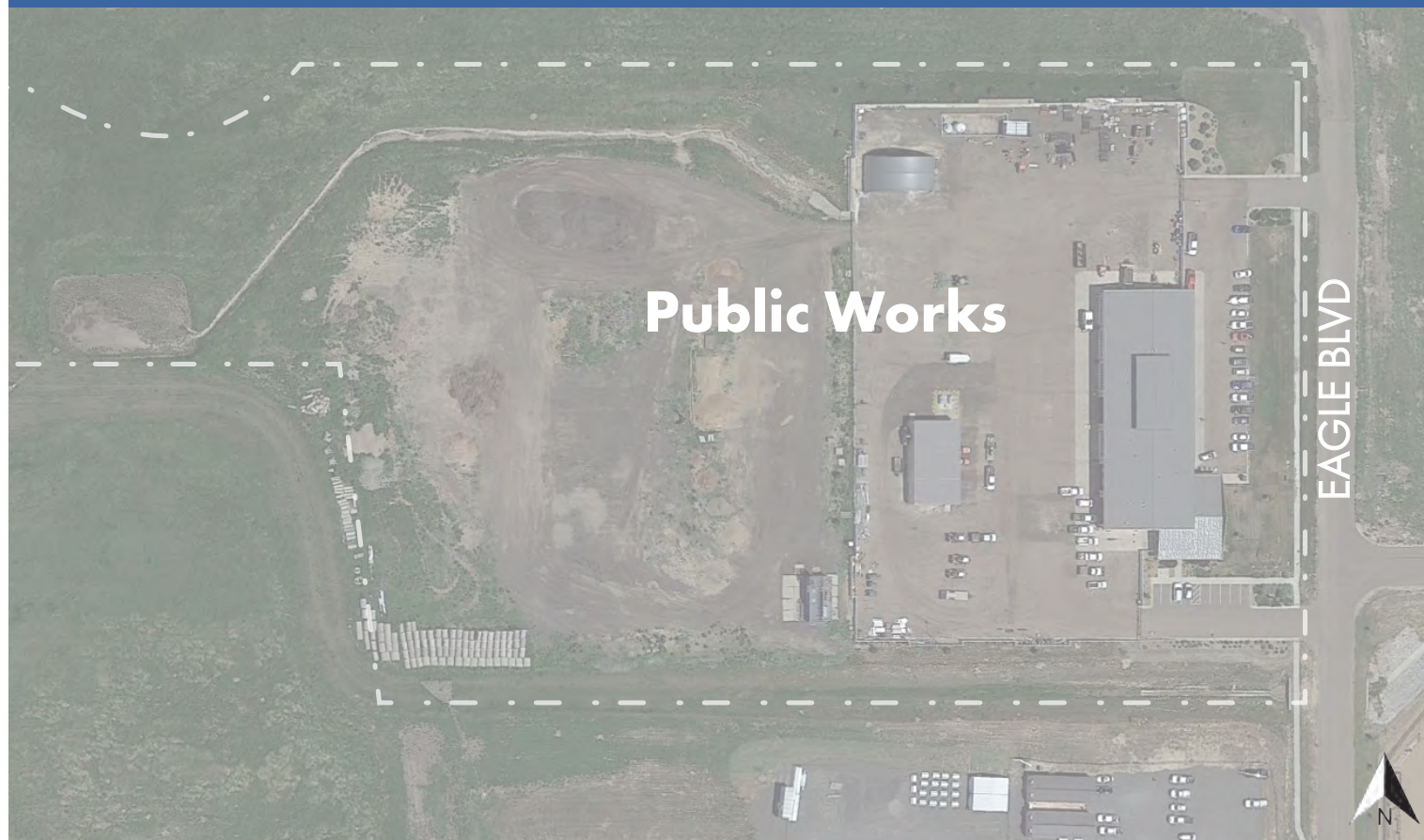
Public Works Site
