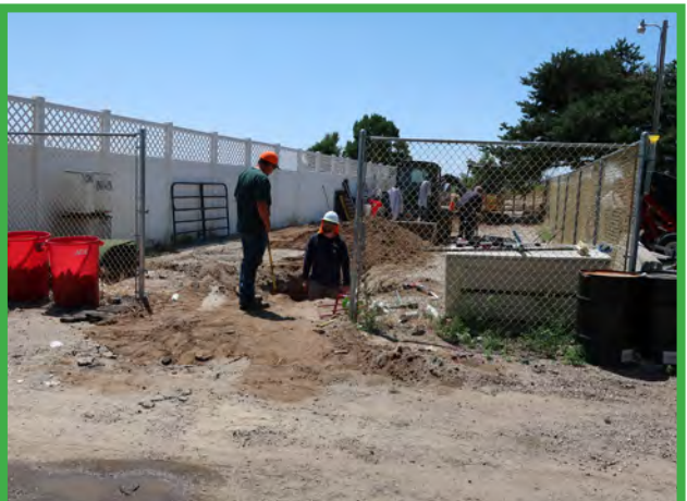
New Golfcart Fleet Storage Under Construction
