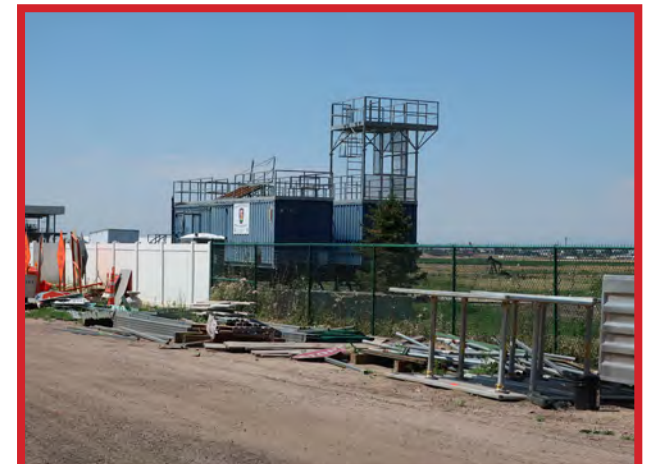
Inadequate Indoor Storage
