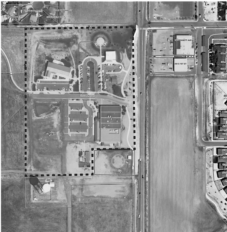
Bennett Town Infrastructure Improvements / Water Tower / Town Hall, 207 Muegge Way, Bennett, CO 80102 Completed date n/a, Project cost $22 M total (Infrastructure package unclear total facility buildout for Town Hall alone).
