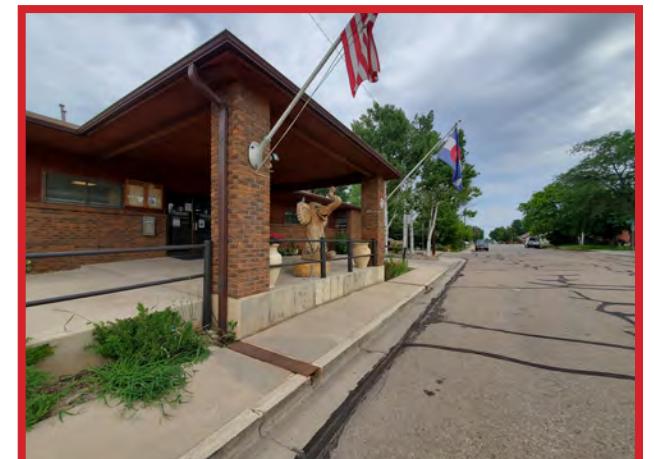
Hard to Find Town Hall Entrance with Unmarked Parking
