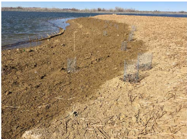
Hunters Overlook Shoreline Habitat Restoration (2019): Bioengineering and wetland restoration to restore shoreline after creation of new 40-acre lake.
