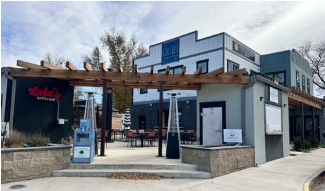
This building at Fifth and Elm Streets integrated the historic patterns of lap siding and windows common in Frederick during its peak as a mining town Credit: RICK
