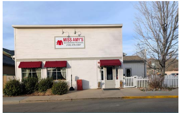
The building, at Fifth and Elm Streets, used horizontal lap siding and vertically oriented windows to mesh with the historic architecture patterns in Downtown Frederick Credit: Town of Frederick
